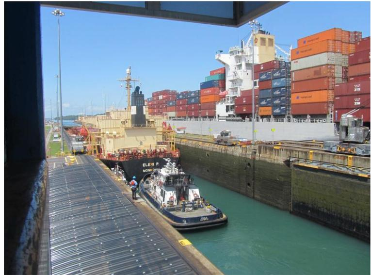
through the locks as the ships move from the level of Gatun Lake down 87 feet to sea level. So tight is the clearance on either side that the huge ships are only 12-15 inches from the walls.
